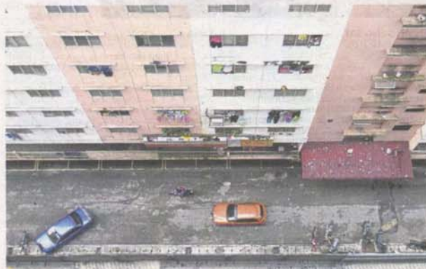
The 'High Rise Security and Safety Manual' touches on security, residents, vehicles, non-residents and emergencies with a proposed by-laws guide for flats. — Filepic
